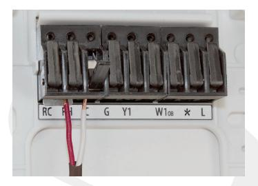
**<u>Attach Wiring</u>:** To insert a wire into a terminal, flip up the locking tab and slide the wire into the socket directly above the corresponding label. Insert each wire as required for the desired appliance. Once each wire is inserted, flip the tab down to lock it in position. Pull gently on each wire after locking the tab is closed to be sure the wire is secure.
