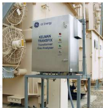
Online DGA monitoring all 9 fault gases plus oxygen and moisture
