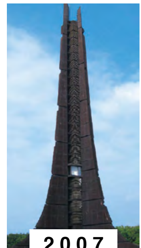
Fuente: Secular changes of appearance of the Hokkaido Centennial Memorial Tower (Sapporo, Japan) employing Cor-Ten steel. Imagen cortesía de Nippon Steel.
