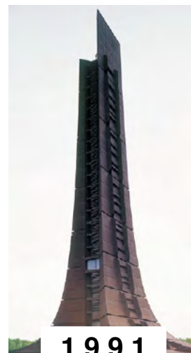
Fuente: Secular changes of appearance of the Hokkaido Centennial Memorial Tower (Sapporo, Japan) employing Cor-Ten steel. Imagen cortesía de Nippon Steel.
