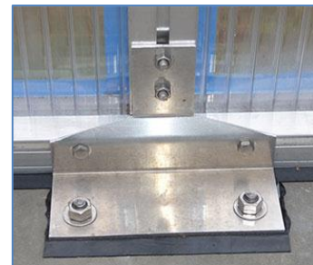
Isolation membrane beneath floor profile and mounting bracket
