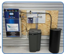
The anolyte generators produce the disinfectant through an electrolysis process using salt and water. This technology ensures employees always have the necessary cleaning solutions on hand and that all facilities are properly and frequently cleaned, without exposing individuals to toxic chemicals. Once installed, a generator produces a 500 ppm HOCL solution for as low as \$0.04 per gallon.
