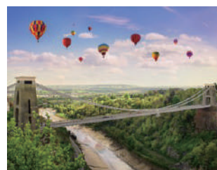
▲ Clifton Suspension Bridge
