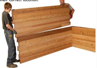
Note: Extra care is needed when placing the upper control panel wall in place. For modular saunas, the controls are typically on the same side of the wall of the heater. Extra care is required to ensure the thermostat capillary line is not crimped or damaged during the installation process.
