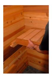
Step 9: Wall bench brackets are preinstalled and benches are pre-built. With the appropriately labeled bench, insert one end on top of the first bracket with the opposite end at a higher elevation. Once the first end is in place drop the opposite end down onto the bracket. If it is a tight fit, use the rubber mallet to drop in place.
