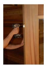
Step 7: Once in place, and the door is plumb, fasten the door/door jamb to the wall with supplied screws THROUGH THE HINGE
