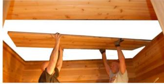
Step 5: insert ceiling panels. All ceiling panels rest on pre-mounted ceiling trim boards. Once in place, make sure ceiling panel seams are tight, then lock in ceiling panels with supplied screws. The ceiling panel screws holes are pre-drilled and located along the top edge of both side panels.
