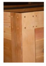
Step 11: All interior and exterior trim pieces are labeled and ready for mounting. They can be brad nailed into place. The exterior trim can be fastened with supplied screws on the corners (as shown above). Plug the holes with the supplied cedar dowels for a beautiful finished look
