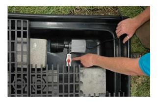
7. Place the mesh over the grating; cut a hole in the mesh for the tubing.
