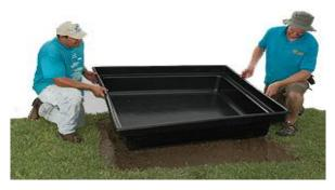
3. Backfill soil around the box packing in firmly.
