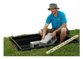
6. Place 2-3 cinder blocks (depending on the piece) in the middle. For light pieces place the grating on top of the cinder blocks. Heavy pieces require several cinder blocks and must sit directly on the blocks with the grate cut away to go around the piece.
