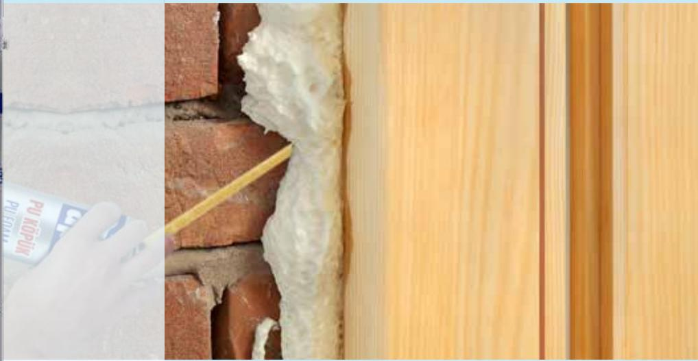
Apel Safety Valved Foam is a polyurethane based, single component, moisture-curing, installation and insulation foam which is used in fixing door and window frames on constructions.
