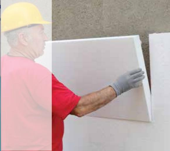
Apel Adhesive Foam is a polyurethane based, single component, moisture curing gun-foam that is used to bond styrofoam, XPS, EPS insulation panels.
