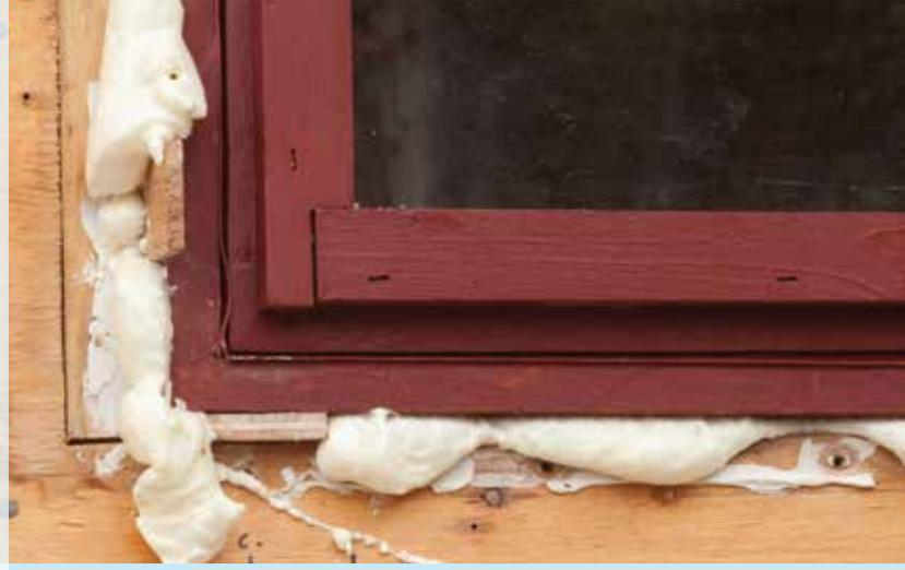
Apel PU Foam is a polyurethane based installation and insulation foam which is used in fixing door and window frames in constructions. Excellent expansion and gap filling properties and solid rigid form after curing make the foam choice of professionals.
