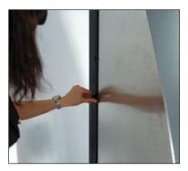
**STEP 6**Insert the sides between the units and rails, starting at the top, clamping them tightly once in position.
