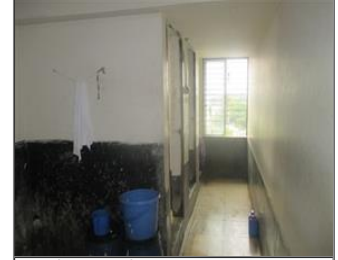
Photo of the sanitary facilities Toilet.JPG
