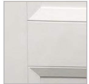
chamfered connection of rails and stiles
