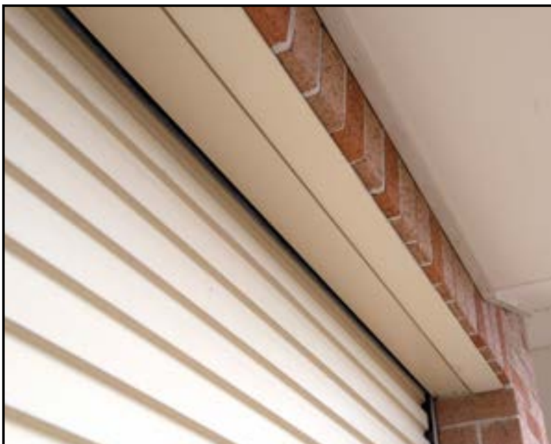
Top seal complete installed view from outside
