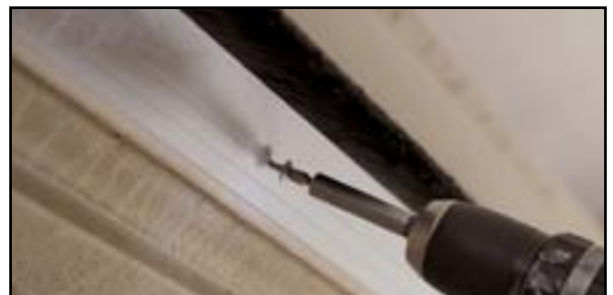
Fixing seal to the roller door
