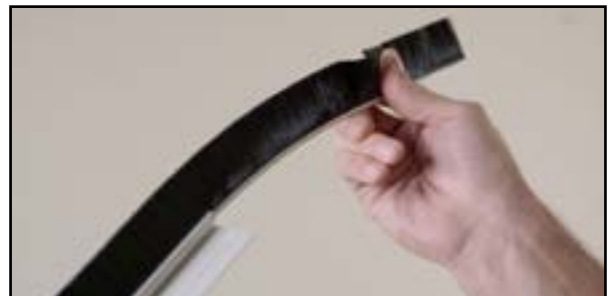
Capture brush into the aluminium carrier
