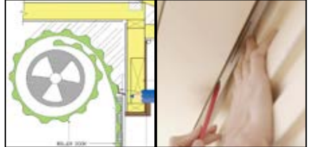
Marking the ridge on your roller door for position
