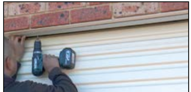
Pre drilling pilot holes
