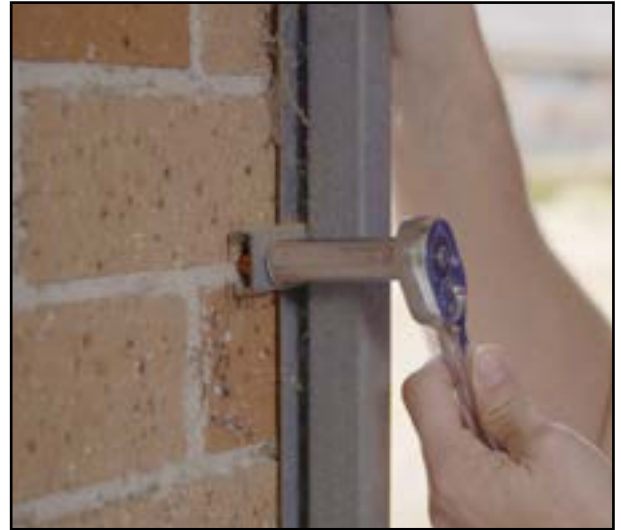
Loosen guide lug bolts on guide tracks SLIGHTLY
