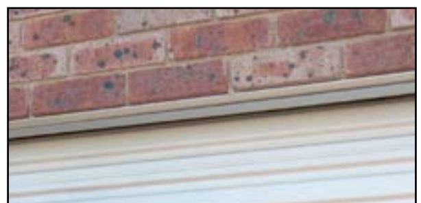
Top seal completely installed view from outside
