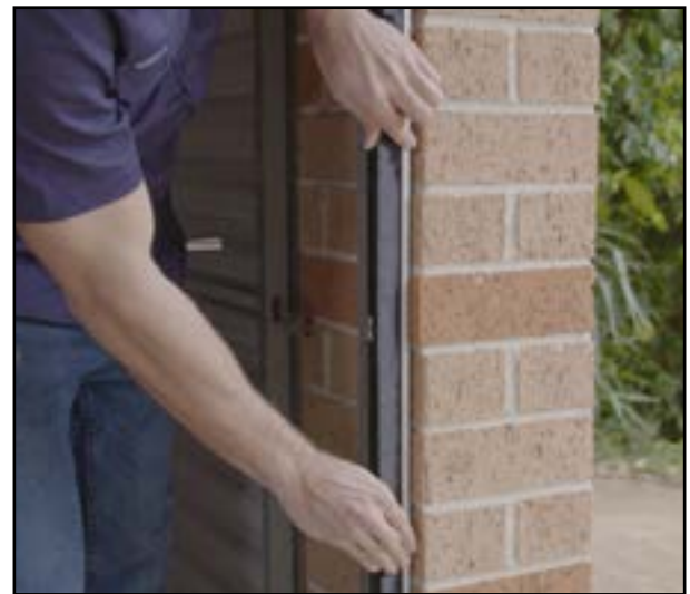
Insert seal between guide tracks and wall
