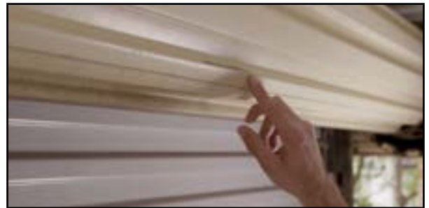
Finding the marked position from inside your garage
