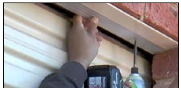
Fixing seal to the lintel
