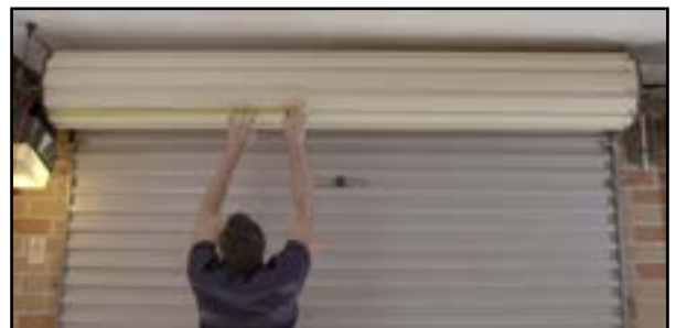
Measuring for fit to door (FTD)
