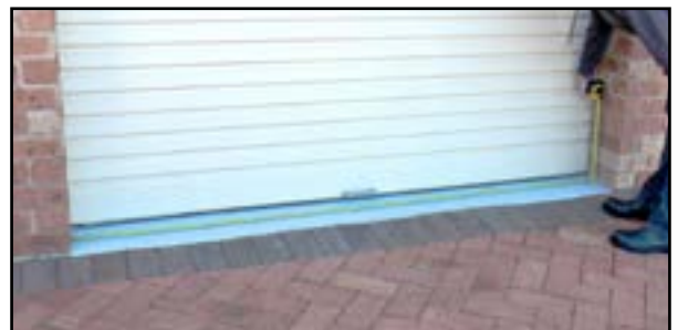
Measuring for fit to lintel (FTL)
