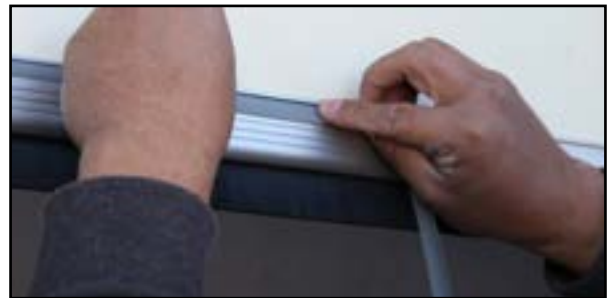
Figure 11. Inserting cover strip
