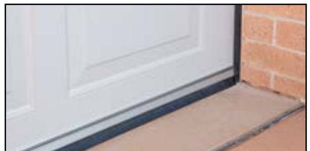
Figure 12. Cobra seal installed with no exposed gaps
