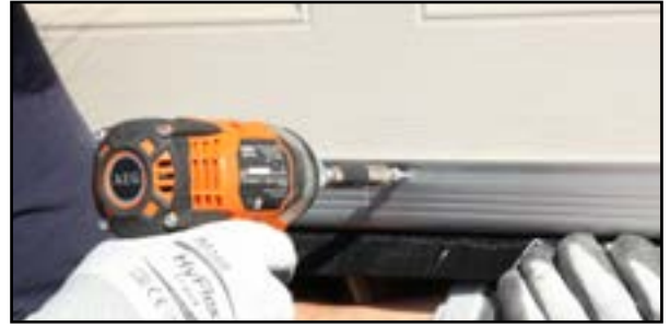
Figure 8. fixing joining lengths
