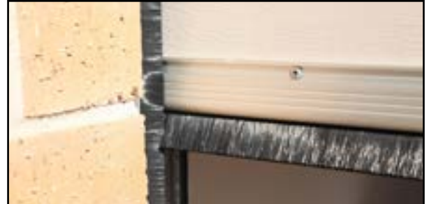
Figure 6. Affix Cobra seal from one end to the other
