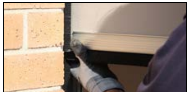
Figure 5. Inserting notched end in position
