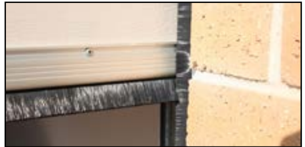
Figure 9. Cobra seal fixed to other side
