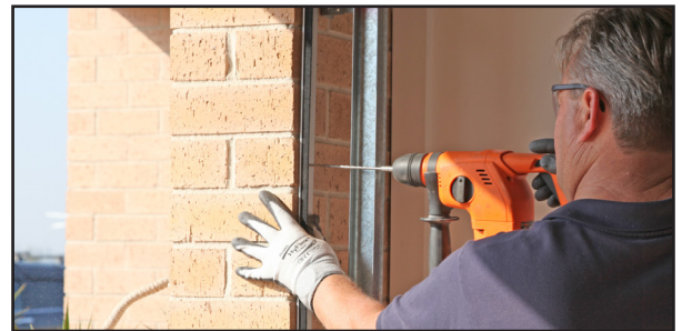
Pre-drill carrier and drill masonry
