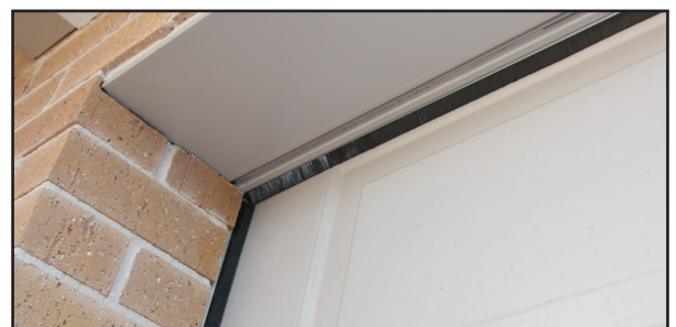
Seals from outside the garage door
