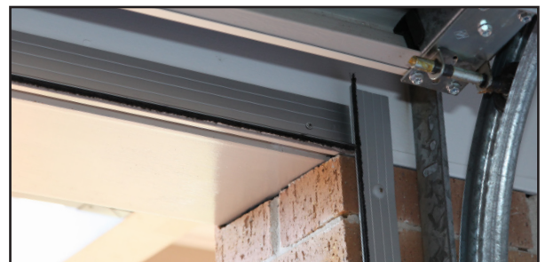
Seals installed from inside garage
