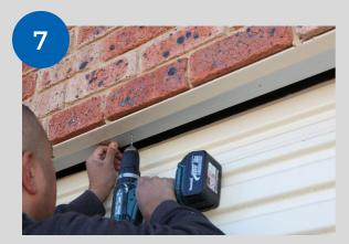
Pre drill holes into the carrier along the length at 300mm intervals, beginning and ending 50mm from either end.
