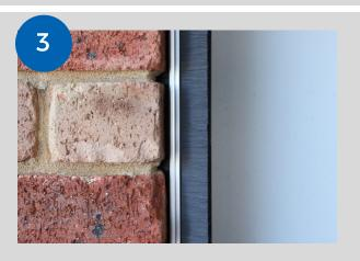
CAPTURE the side seals in the aluminium extrusion by withdrawing 100-150mm of the brush then creating a gentle sideways radius bend in the metal backing spline, the brush should be reinserted back into the aluminium and tested to see if it can be easily removed by hand.
