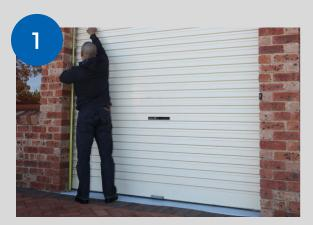
Measure the side seals first, allowing the seal to run up past the top of the opening by at least 50mm.
