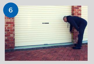
Measuring the width of the opening, cut the top seal aluminium to length after sliding the bristle brush back first. After confirming the aluminium is the correct length, cut the brush to match, using pliers or side cutters only.
