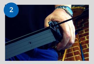
If the seals must be cut, mark the length then PULL the brush back, away from where the aluminium is to be cut. Cut the aluminium to length. Slide the brush back and cut to the same length as the aluminium using PLIERS or SIDE CUTTERS ONLY.
