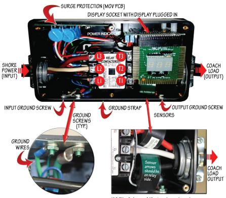
**NOTE:** Only one (1) wire through each sensor. Black wire goes through curent sensor (with green tape) to T1.
