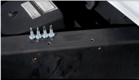
Fig. 4 – Pilot holes shown with included self-tapping screws.
