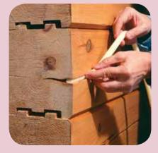
Install backer rod into a clean, stained check to the appropriate depth. (See Fundamental Application Guidelines.)
