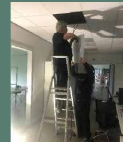
INSTALLATION OF LED LIGHTING
