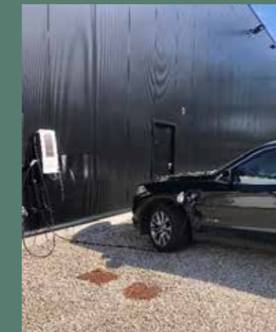
INSTALLATION OF CHARGING STATION
