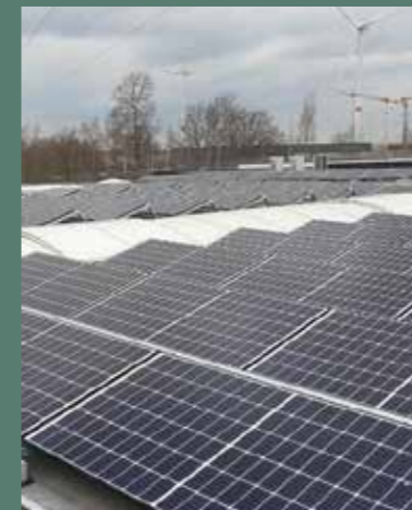
INSTALLATION OF SOLAR PANELS
