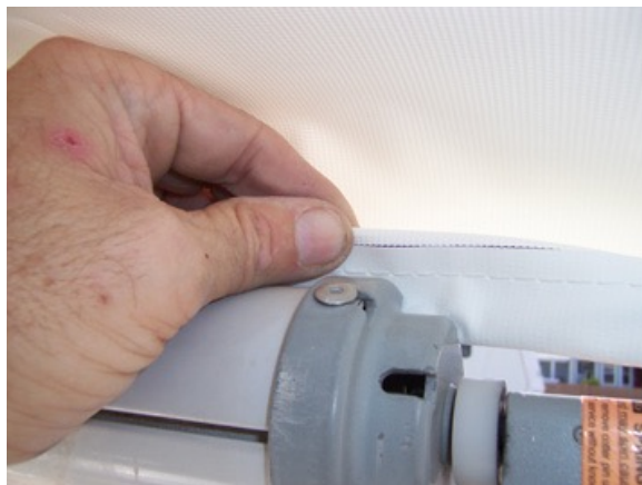
Feeding Fabric into Roller Tube
