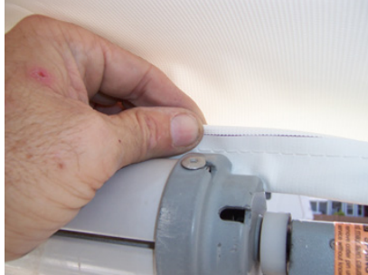
Feeding Fabric into Roller Tube
