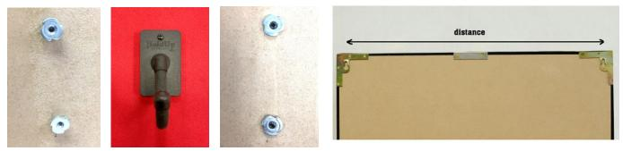
**Step 6:** To hang the cabinet on the wall, simply position the cabinet over the top 2 screws and align with the holes of the Tear-Drop brackets. Slide down the case and have it rest on the brackets. Now you are ready to use the cabinet to display your items, test fit the hanger with item again and adjust the hangers if need.
