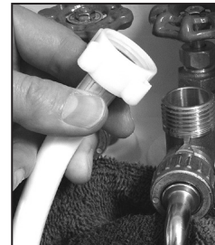
Remove intake hose and re-attach
