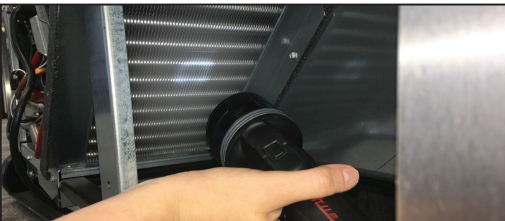
Fig. 4. Verify all blockages have been removed.
