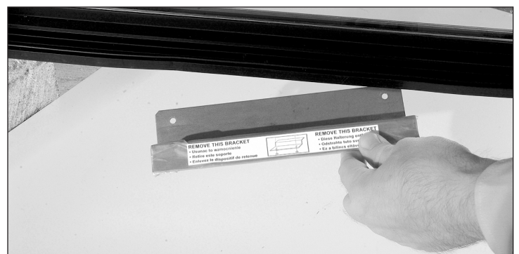
Fig. 2. Remove the glass swing door shipping bracket, if so equipped. Do not discard.
