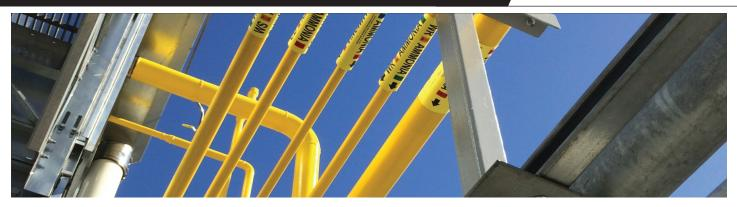
Bulletin 114 was developed and published in 1991 as means to establish uniformity among ammonia refrigeration users and practitioners in identifying refrigerant piping. The basis of the guidelines was ANSI Standard A1.1-1981 "Scheme for Identification of Piping systems". In 2007 ANSI A13.1 was to indicate that orange backgrounds, rather than yellow should be used to indicate toxic and corrosive fluids (i.e. Ammonia). Bulletin 114 was recently updated in 2014 to reflect this standard.
