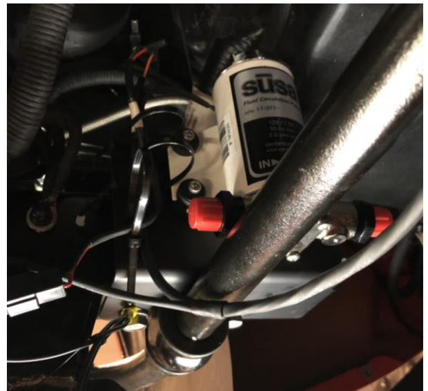
Differential Pump Installed with Ground Lug
