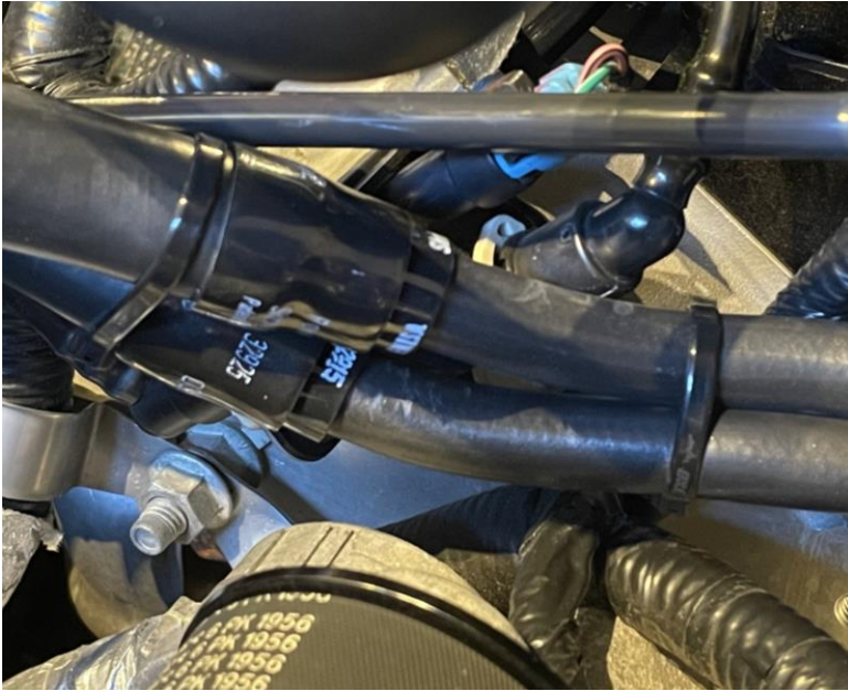
Ty-wraps securing the hoses together.
