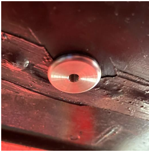
Fully Installed Stainless-Steel Boss
