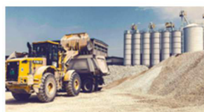
Run Hours Monitoring
