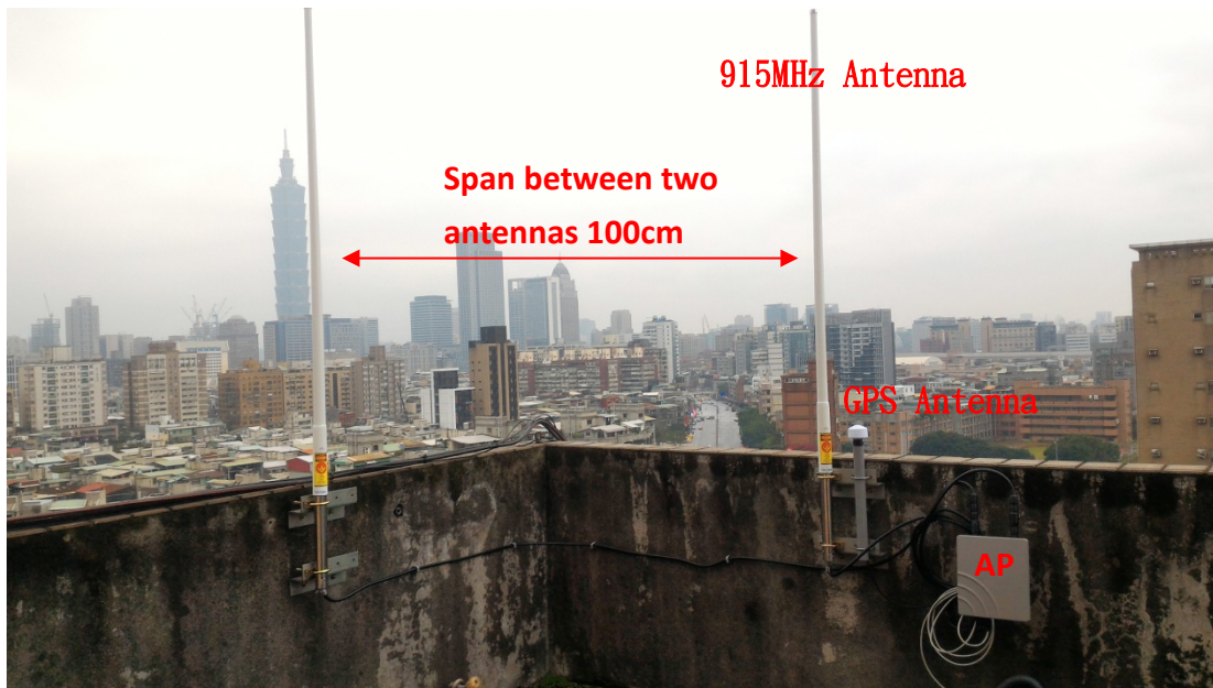
Figure 21 Actual View of a Wall-mount Installation
