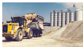
Run Hours Monitoring
