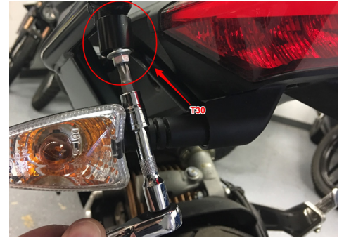
Figure 13. Secure Top Rack Turn Signal Support
