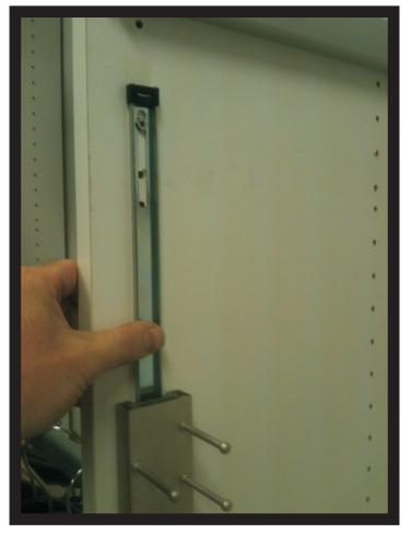
Slide the rail out and let the tie rack hang so that the left mounting hole is under the slot on the glide arm. Insert the first mounting screw.
