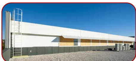
Roof Top Plant Rooms
