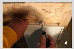
Mount flush to ceiling, wall or other flat surface, although they may also be suspended.
