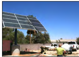
SOLAR PANEL CLEANING
