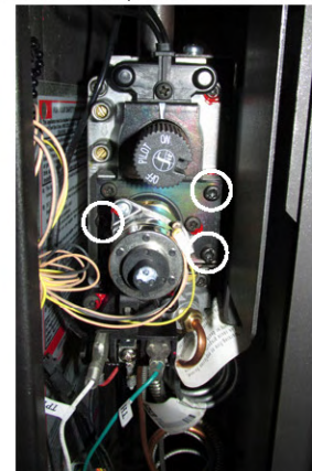
Remove NG Stepper motor and replace with LP Stepper motor
