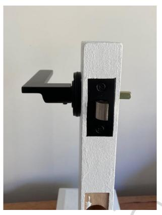
7. Push external handle with sleeves attached on to the spindle that is currently sitting in the latch.
