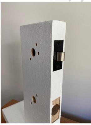
2. Insert latch and fix in with screws.
