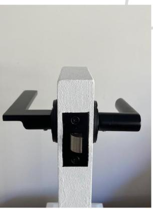
8. Push internal handle over the spindle that is currently sitting in the latch.
