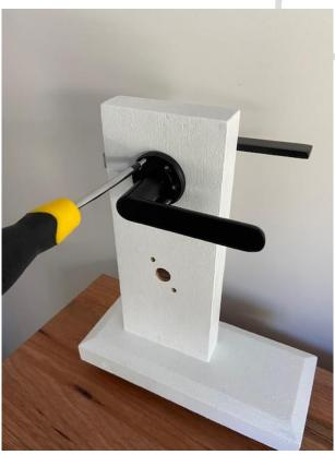
10. Tighten the long fixing screws using a hand screwdriver. Be careful not to over tighten.
