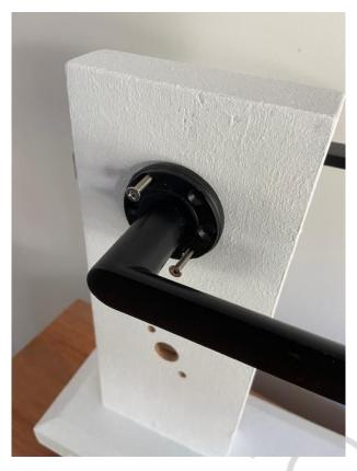
9. Insert the 2 x long screws through the internal handle rose in to the fixing sleeves.
