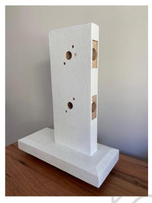
1. Drill holes according to the product template, including checking the latch face into the door so that it sits flush.
