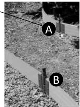
When your desired location is achieved slide out your first stake, flip it around **B** and drive the stake point through the bracket loops and into the ground.
