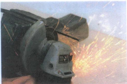
5: Cut the damaged inner shaft
