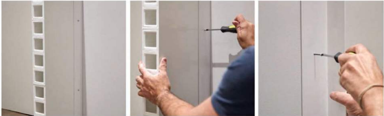
Removing a Finishing Cap using a knife blade
