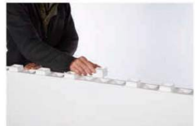
Installing Connector Lugs on top of an EverPanel, in anticipation of installation of another row of panels.
