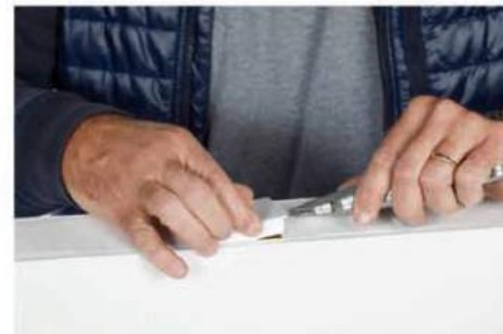
Removing a Finishing Cap using a knife blade
