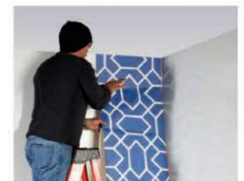
Installing a first section of adhesive backed wallpaper.
