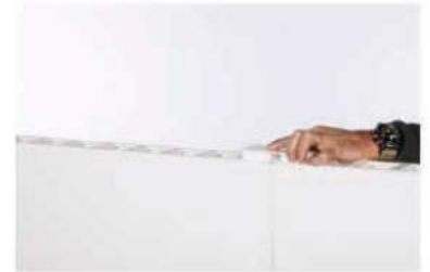
Installing an Inter-Panel Locking Connector on Top of panels
