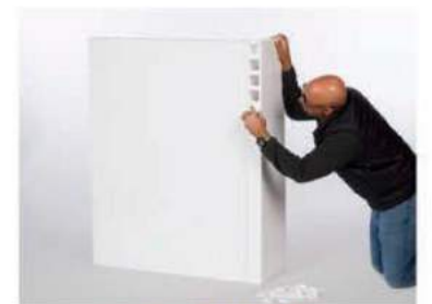
Installing Finishing Caps along the side of a wall
