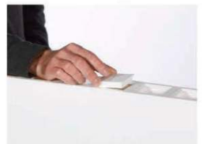
Installing Finishing Caps on an EverPanel
