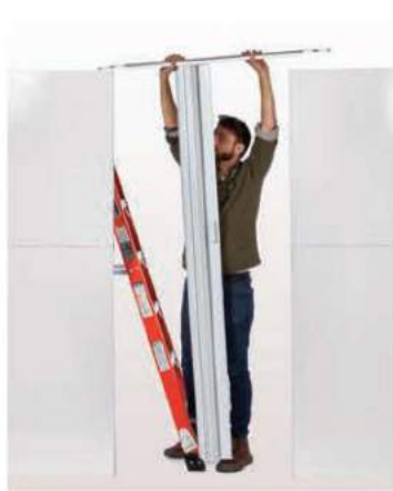
Positioning a Lintel with Accordion Door on top of EverPanels.
