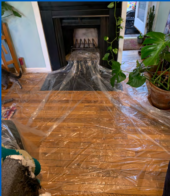
Install sanitary barrier in work area
