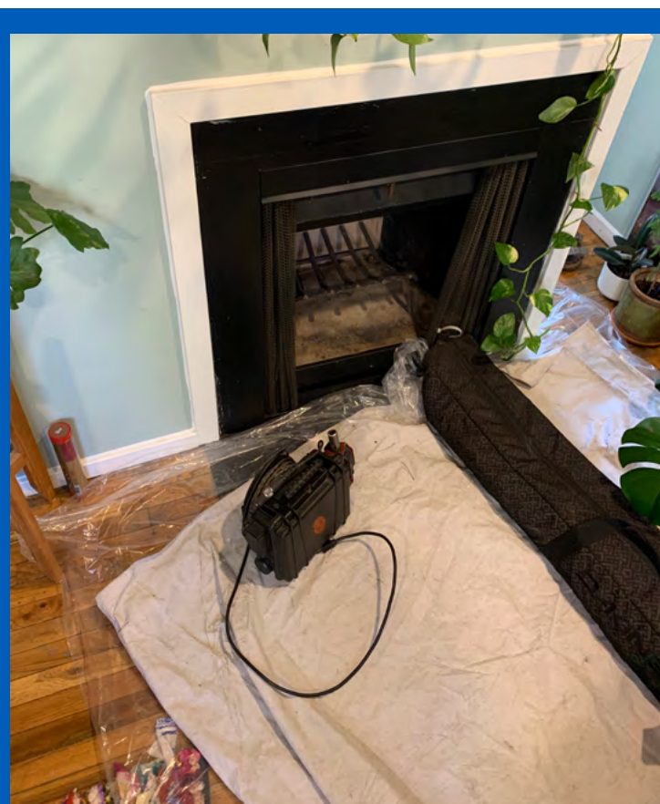
Unsanitized work tarp between work tools and sanitary barrier (new plastic)
