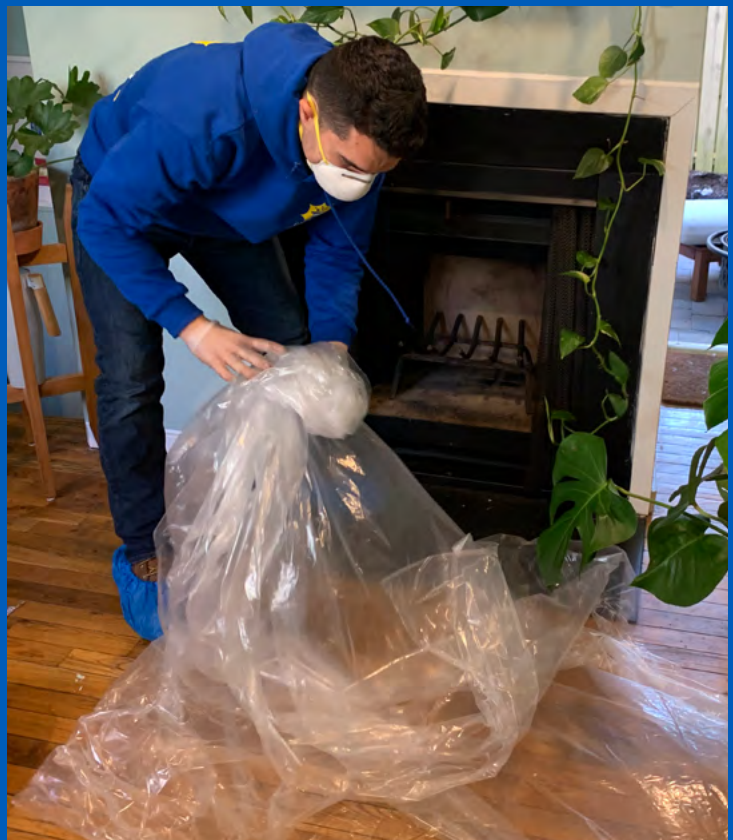
Remove sanitary barrier from the home
