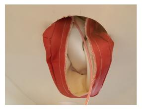
Fold the hood and push it up through the speaker cut out hole. Open the hood out and make sure the flange is sat flat on the plasterboard.
