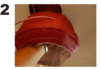
Pierce a hole through the side wall with stanley knife and feed the speaker cable through the hole. Keep the hole to the minimum size required to allow the cable through. In the event of a fire the material expands to seal the hole.
