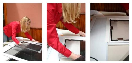
When installing the spline in the corner of the pet door unit, it may be necessary to cut a small diagonal slit up into the screen material in order to relieve the tension on the screen
