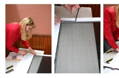
work very well for removing the screen spline or can also vou carefully use a screwdriver at the corner to get started. If using a be screwdriver. careful not to cut into the spline or into slice the finish of the door frame. HINT: Only remove the spline
