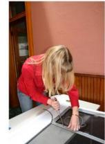
from the outside. NOTE: If there is not enough clearance on the inside frame for the screw heads due to a stationary door or narrow а screen frame, the screen model must be attached from the outside.
