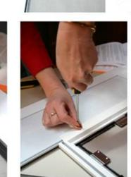
fabric and allow it to be pulled down into the spline frame track. NOTE: Be careful not to cut too far into your screen fabric or you will have a hole at the corner of your pet door. See the picture to the right for a close up of a correctly installed pet door.
