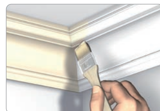
Paint the cornice in the same colour as the wall or ceiling
