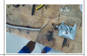
Screw the electrical conduit back into the new motor by screwing the conduit clockwise.
