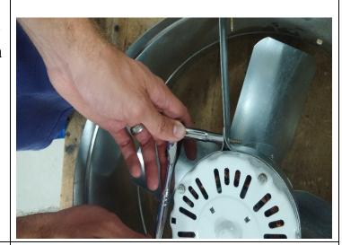
When all three bolts are loosened you will be able to slide the motor out of the motor bracket.
