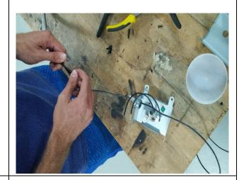
If the wires are difficult to reinstall into the electrical conduit, install a piece of wire into the conduit. Tape your motor wires to the wire you installed and use that wire to pull your new wires thru the conduit.
