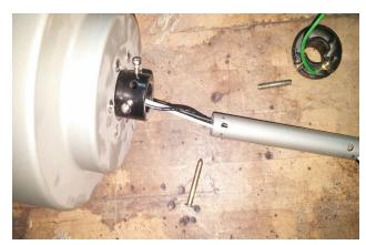
Step 4: Attach the downrod to the motor by installing the pin and cotter pin and tightening the two screws. YOU MUST TIGHTEN THE TWO SCREWS TO PREVENT THE FAN FROM WOBBLING.
